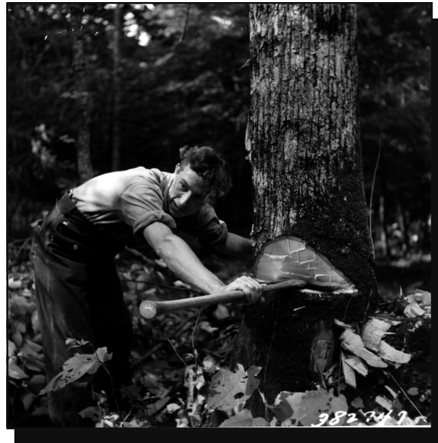
Figure 59—A double-bit ax is being used as a T-square to indicate the direction of fall in this 1939 photo from West Virginia. Today, hardhats and eye protection would be required dress.
